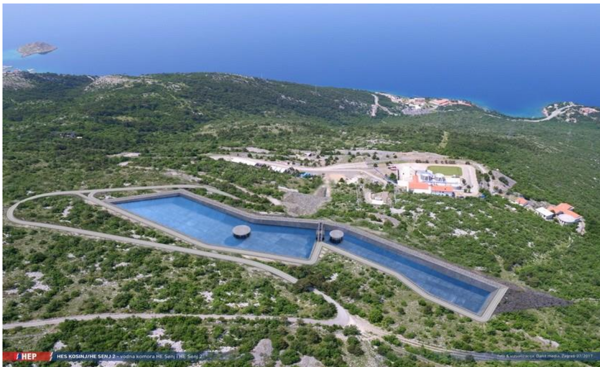
Slika 17: Prikaz HES KOSINJ / HE SENJ 2 – vodna komora HE Senj i HE Senj 2
